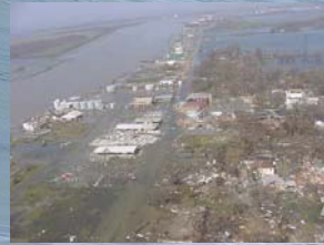
Cameron, LA Aerial View
